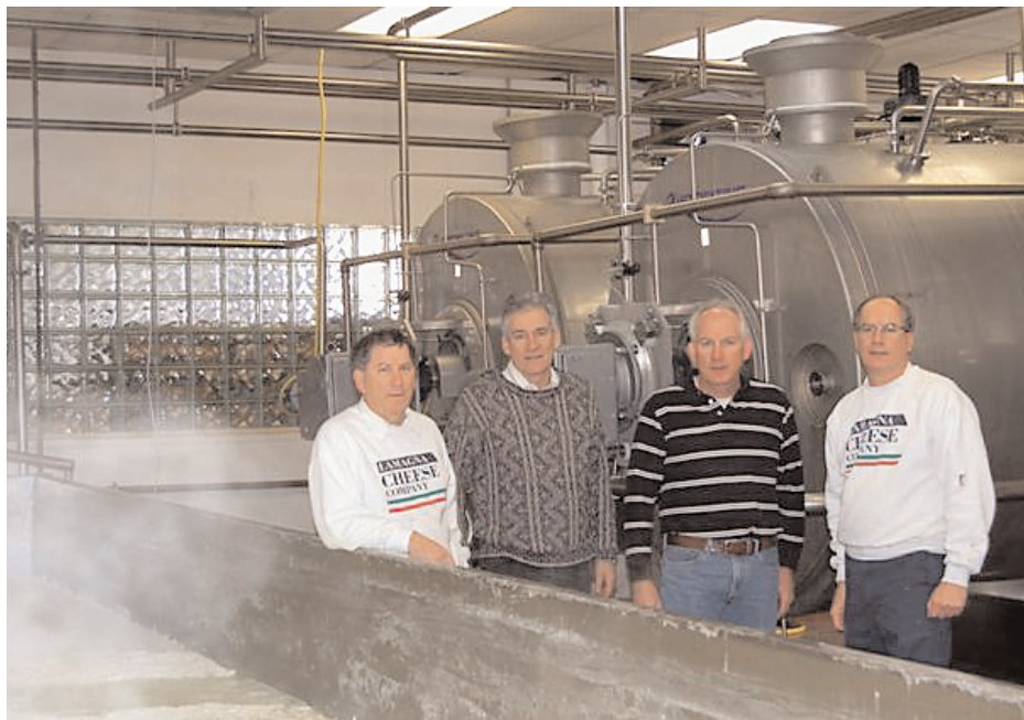
Mike, Rudy, Kirk and Chris Lamagna stand in front of their new Stoelting vats while steam comes off their last open vat. Lamagna Cheese and Stoelting recently design an enclosed vat specifically made for the company’s milk-based Ricotta. The new vats have worked so well, the cheese company is looking to stop production in the open vat entirely.
